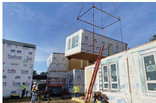
Figure 25: Type 5-over-1 in The Acacia (left) Prefab Construction in Eastmoor (right)
